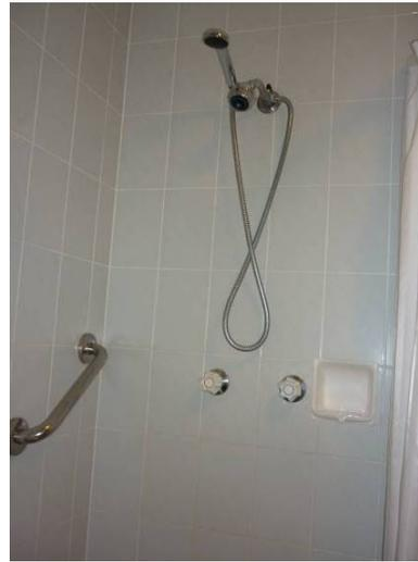
The shower is fitted with a grab rail which is on a slope from 955mm up to 1090mm from the floor. There is an adjustable shower seat provided. The shower has a fixed shower head and a shower head on a rose, which is mounted high, so assistance will be needed to reach it. (as shown) There is no clearance under the sink as there is a cupboard, although the sink is close to the front of the cupboard and it at a height of 800mm. The base of the mirror is 875mm from the floor.
