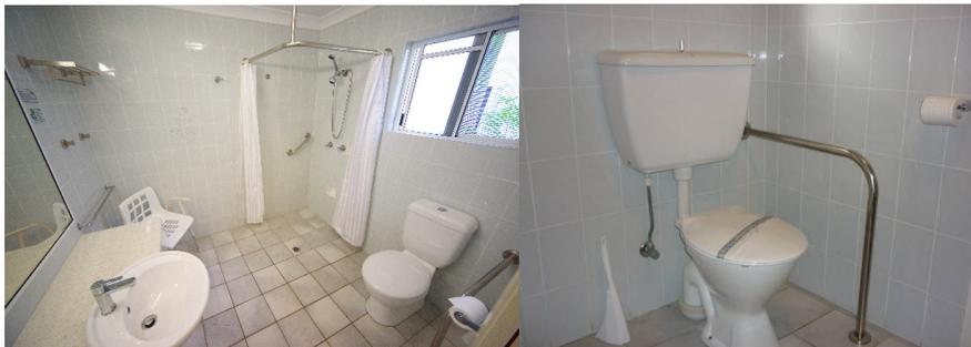
Entry into the accessible shower and toilet is through a sliding door with a clear width of 800mm. The facility is a combined toilet and shower with a dimension of 2380mm long by 2070mm wide.
